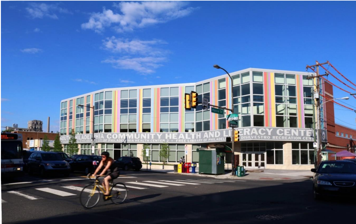
South Philadelphia Community Health and Literacy Center, facing Broad Street. Shows curtain wall for floors 2 and 3, cantilevered entry way, and cantilevered screen wall.
