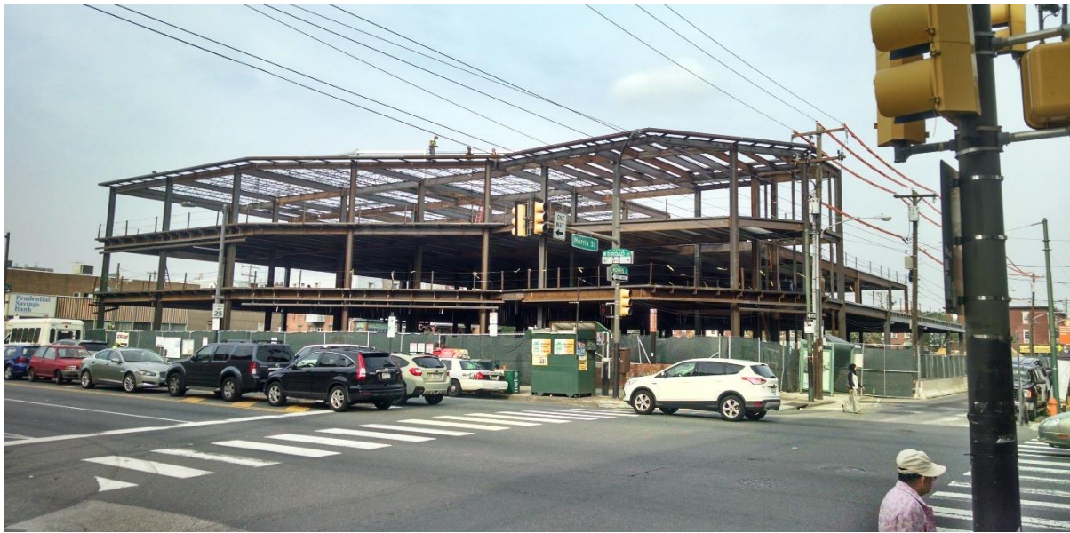
New structural steel framing erected during construction. The use of moment frame connections provided accelerated construction time and allowed for open floorplans throughout the building. (photo ©Keast & Hood)
